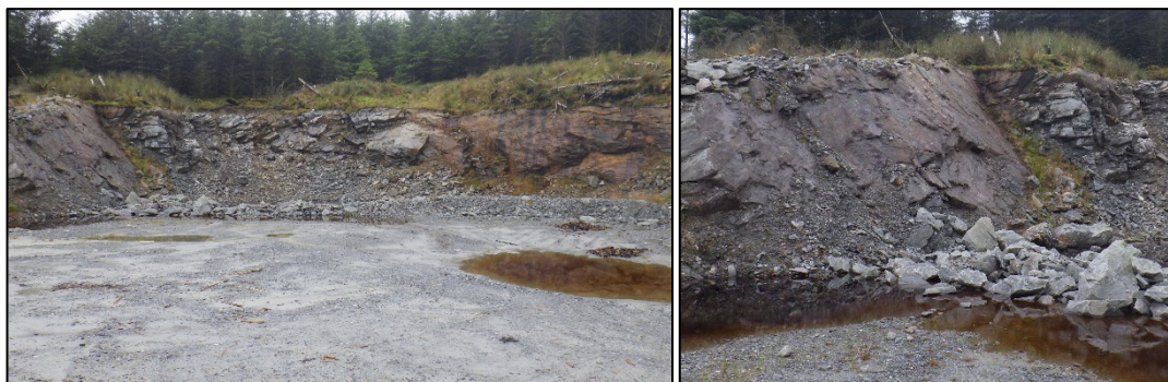
Figure 10.3.F: (a) View of BP5 (FLS) looking N, NGR NR 8935 6217. (b) Close up view of the borrow pit wall.
