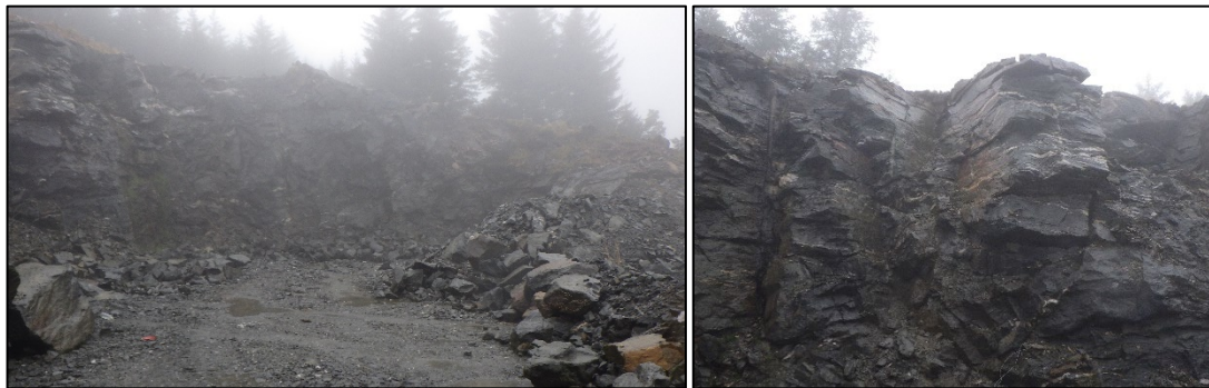
Figure 10.3.E: (a) View of BP4 (FLS) looking N, NGR NR 8774 6239. (b) Close up view of the borrow pit wall.
